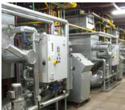
▲ LOI developed Bypass cooling system featuring dual cooler installed in the basement
